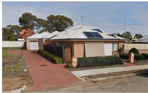
Dawson Street Units
