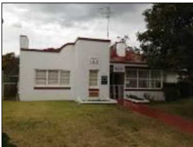
Old Infant Health Building (External)
