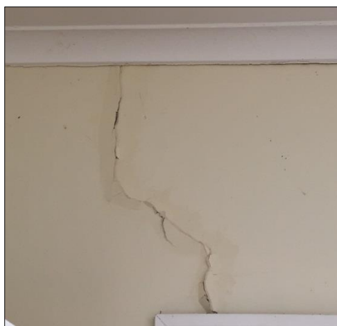
Old Infant Health Building (Internal)
