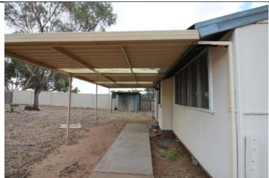
House 23- rear verandah area
