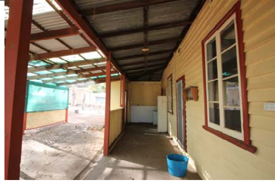
House 24- rear verandah area
