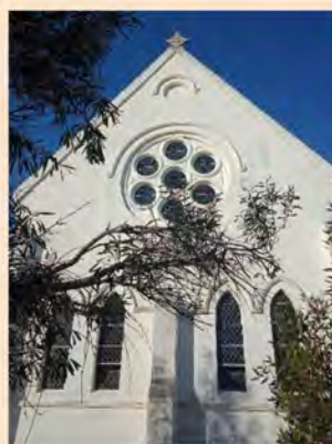
St Mary's Anglican Church Beverley
