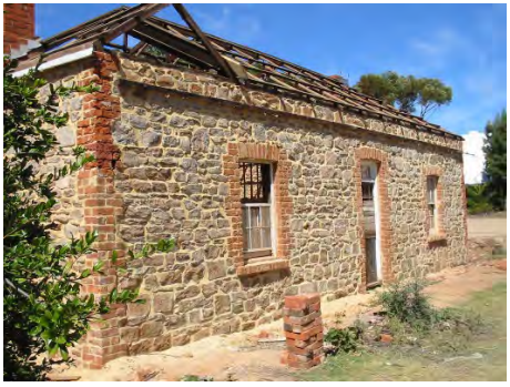
Exposed rafters during renovations
