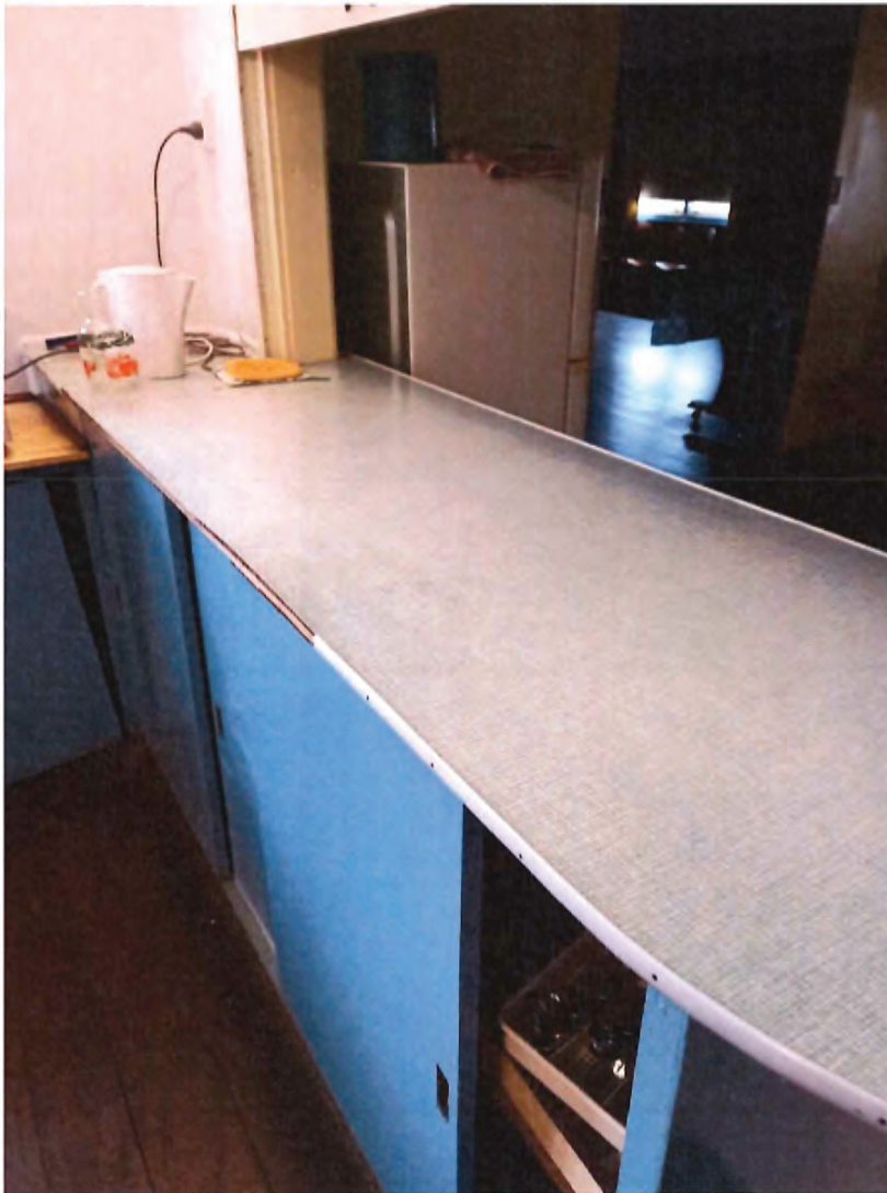
Existing bench tops
